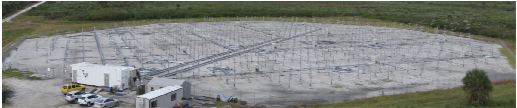
RAPTOR FBS-MST Scalable Mesospheric-Stratosphere-Troposphere 50 MHz Radar Wind Profiler. Installed for NASA Kennedy Space Center in 2014. Shown configuration uses 640 Yagi elements, 150 m diameter antenna, and 320 kW peak transmit power. Typical range is 20 km.
