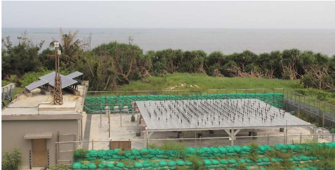
Figure 2 – RAPTOR Stratospheric-Tropospheric Radar Wind Profiler Installation on Dongsha Island
