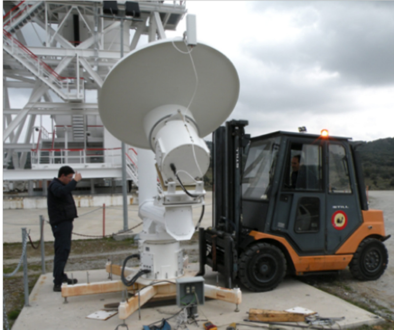
Figure 1. The AWVR installed at DSS-55.
