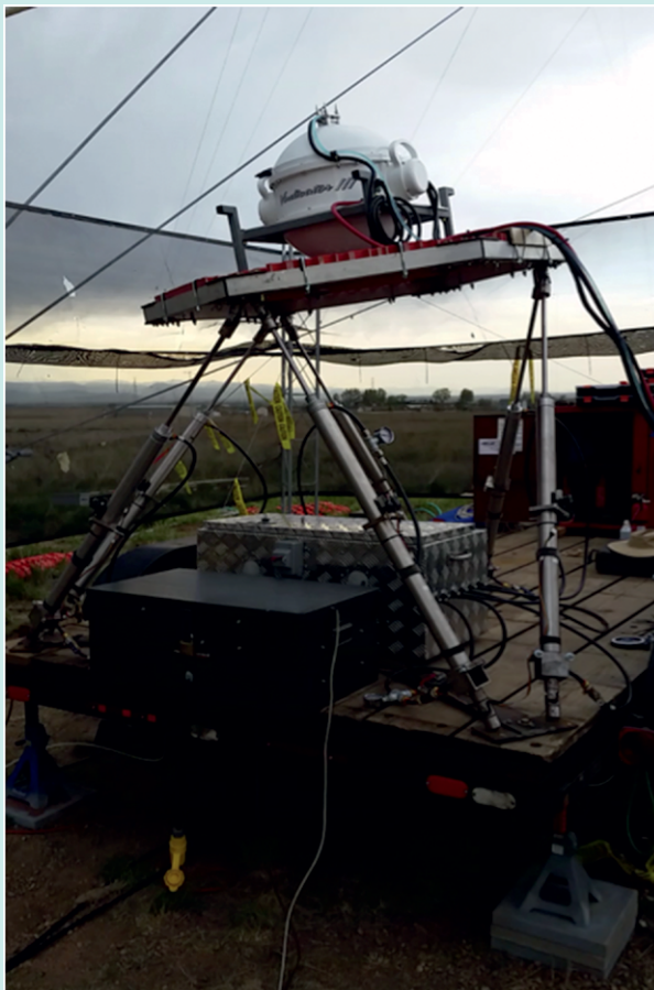
FIG. SBI. The UMBC pneumatic Stewart platform at the BAO with a Vindicator III mounted. The guy cables of the BAO can be seen in the background.
