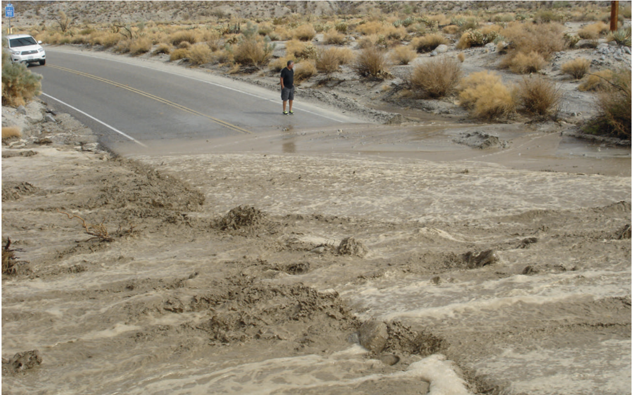
FIG. 8. Flooding across Highway 78 in San Diego County, California, 22 Jul 2013. [Photo credit: NOAA]
