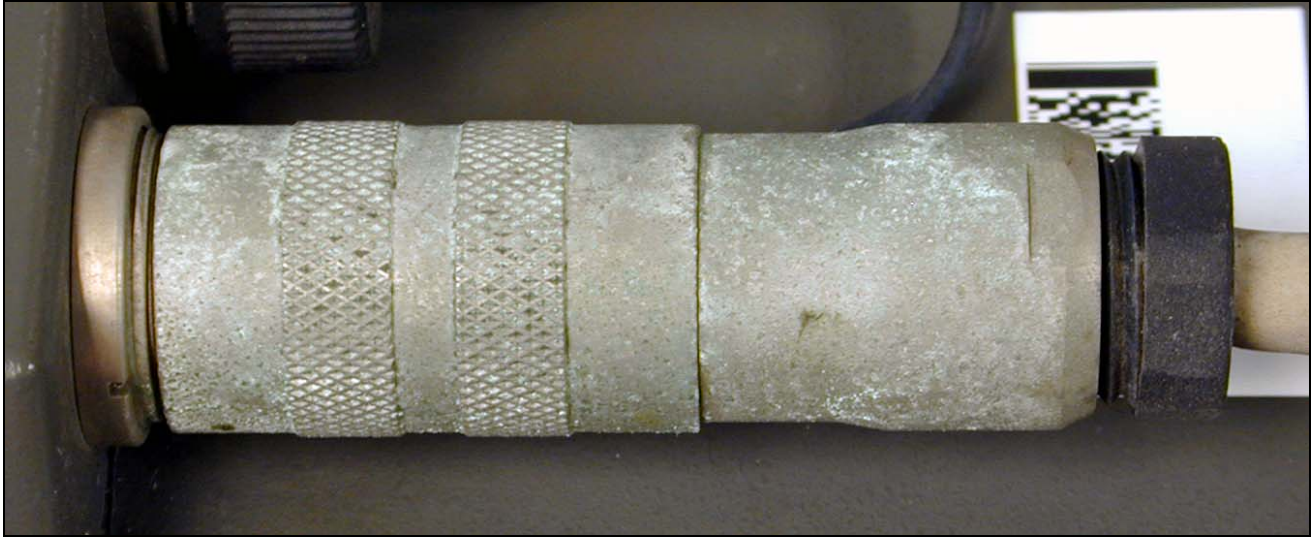
Figure 11. IRT cable connector housing showing corrosion and oxidation.
