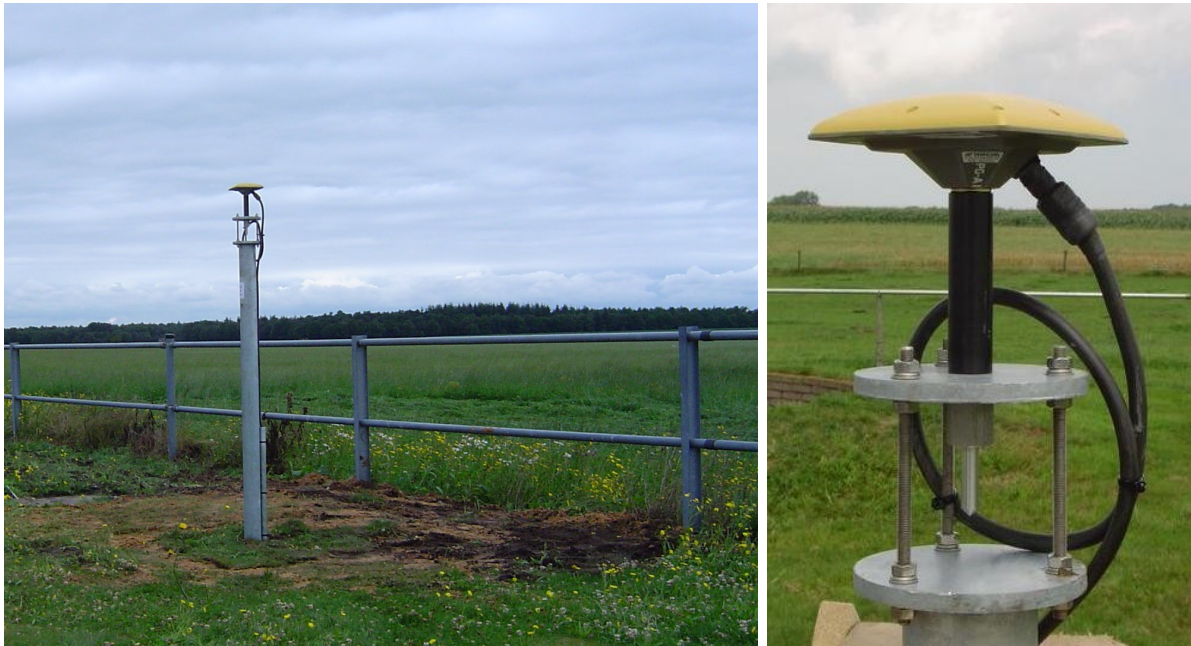
Figure 1.4: GPS antenna installed on a weather station in the Netherlands. The receiver is located in a nearby shed.
