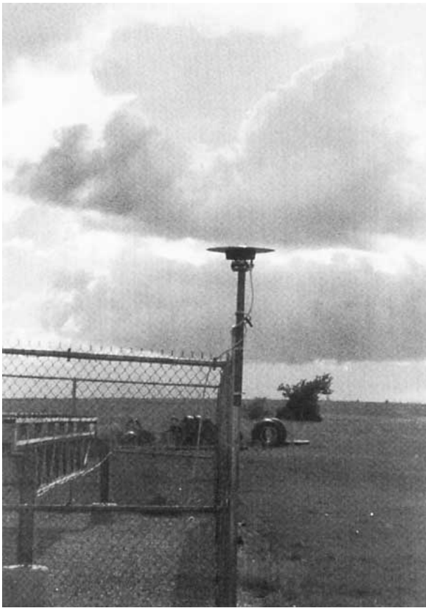
FIG. 4. Photograph of a GPS receiver antenna mounted on the perimeter fence of a NOAA wind profiler. The diameter of the antenna ground plane shown is ~50 cm.
