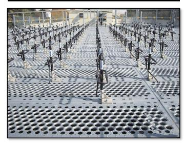
Yagi antenna elements deliver easy installation and maintenance. Components are user replaceable in the field for maximum uptime and improved data quality.
